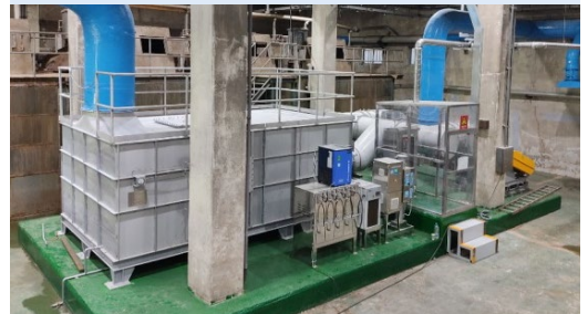
Busan OO Sewage Treatment Plant
