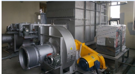
Busan OO Sewage Treatment Plant
