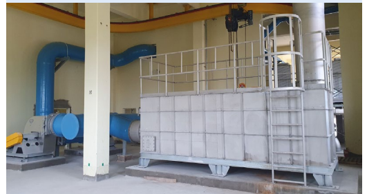
Ulsan OO Sewage Treatment Plant
