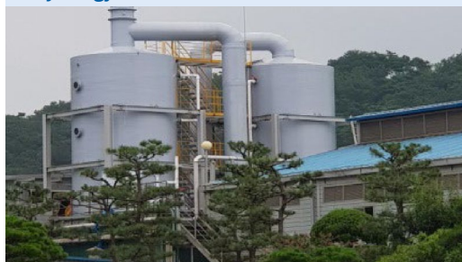
Gyeongju OO Wastewater Treatment Plant
